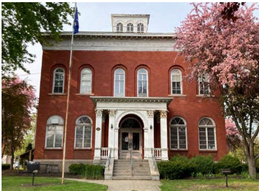
Brisbane Mansion— 10 Main Street Reuse Analysis completed to determine a utilization plan in preparation of the City Police Department moving into their future new facility.
